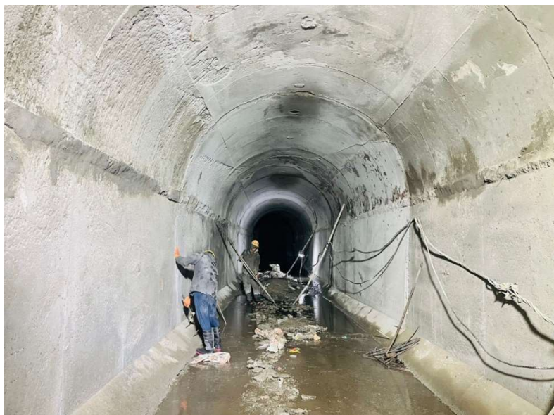
Face 2: Full lining work in face 2 completed
