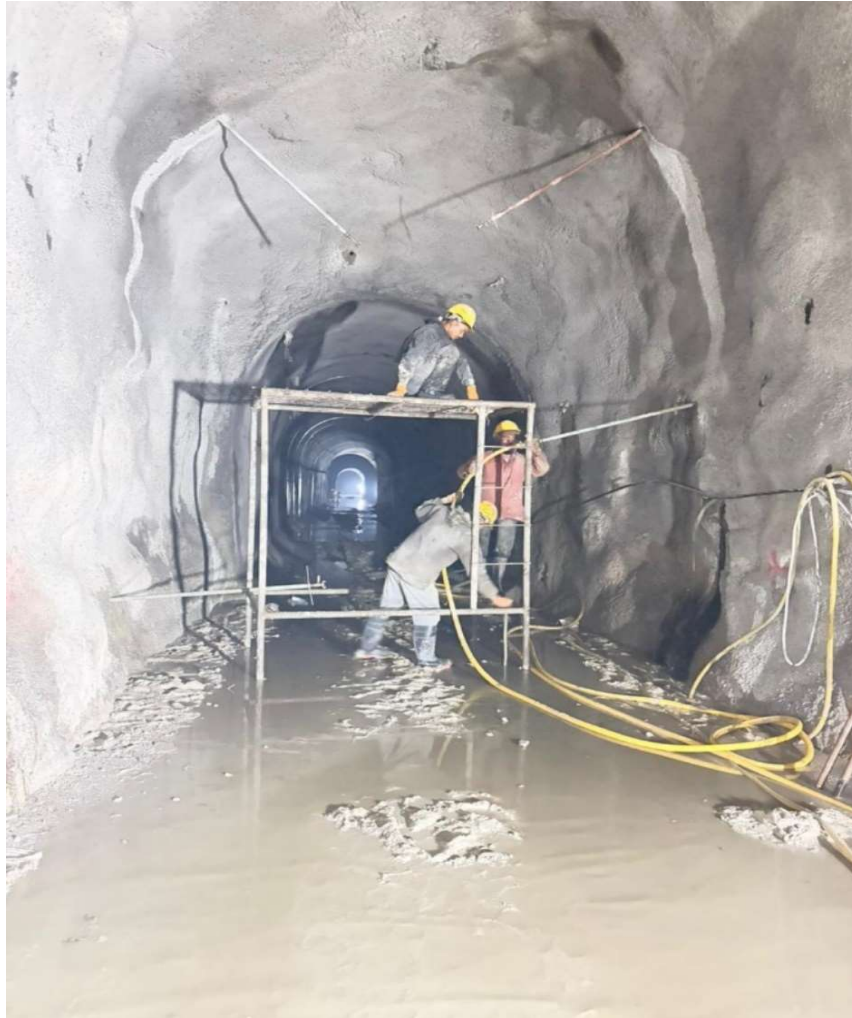
Consolidated grouting work at Face 2
