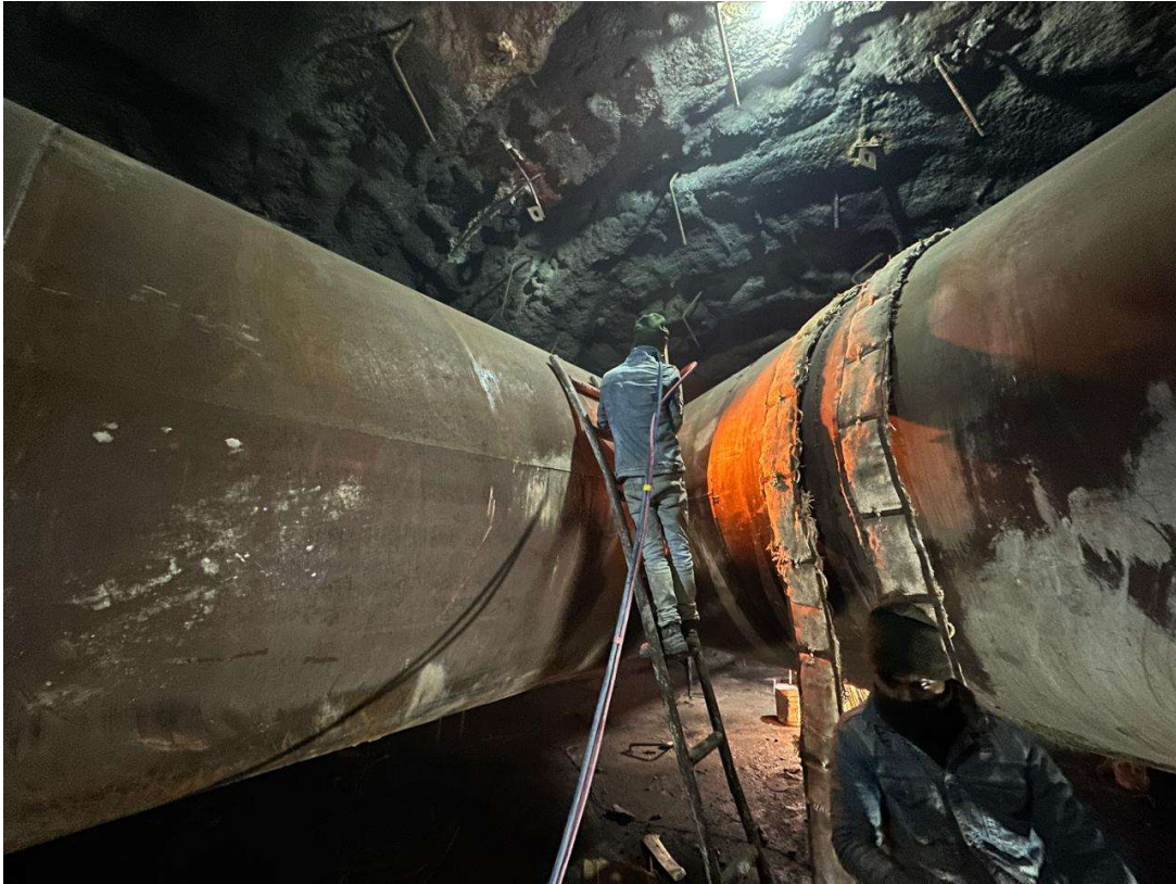
Pipe Installation work at T Junction
