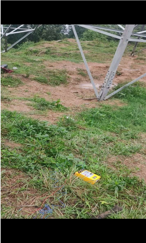
Measuring Transmission Line Tower Footing resistance
