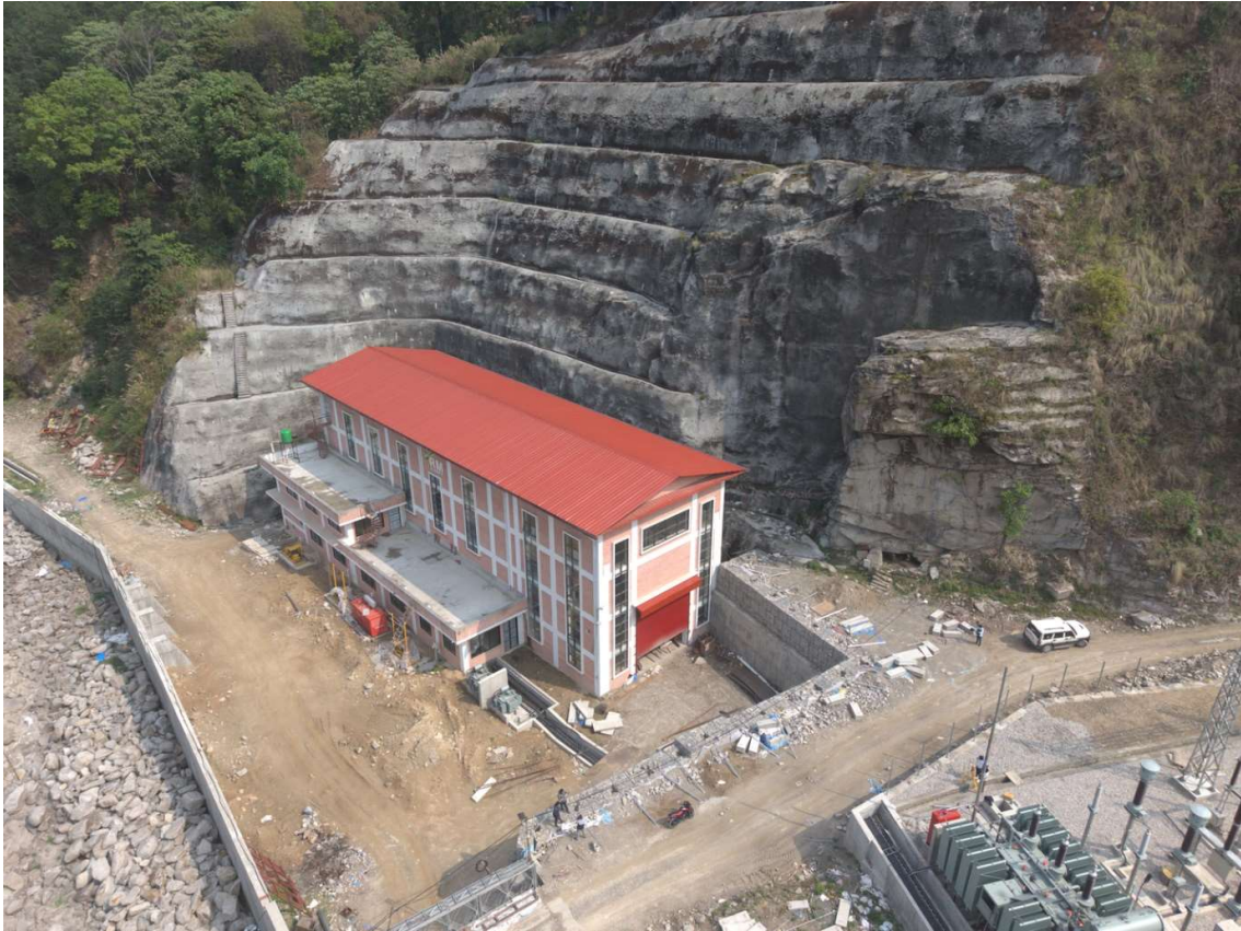
Figure: Overall View of Powerhouse
