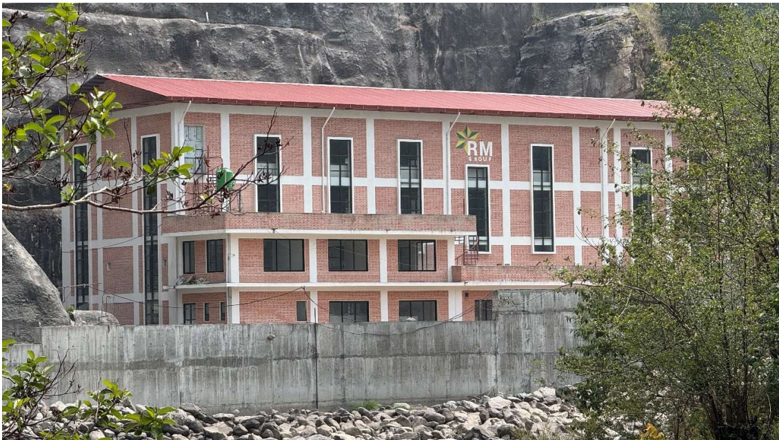
Power House of K2HEP
