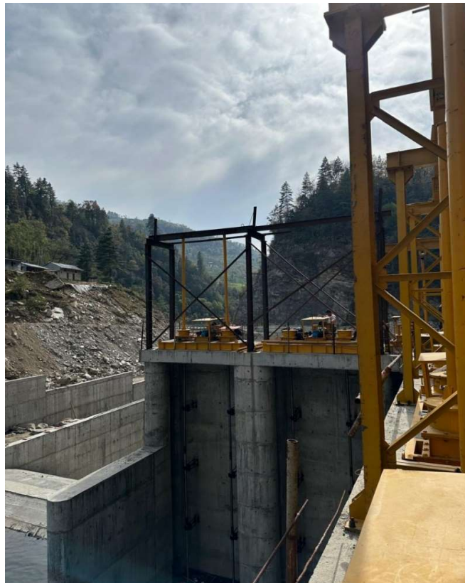
Under Sluice Gate
