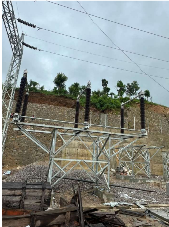
Bypass isolator installation
