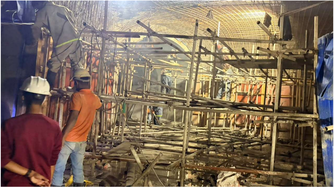
Junction Rebar Work
