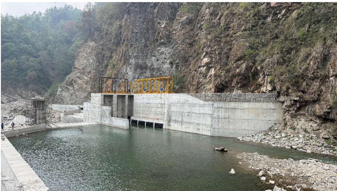
Overall, View of the Headworks Area
