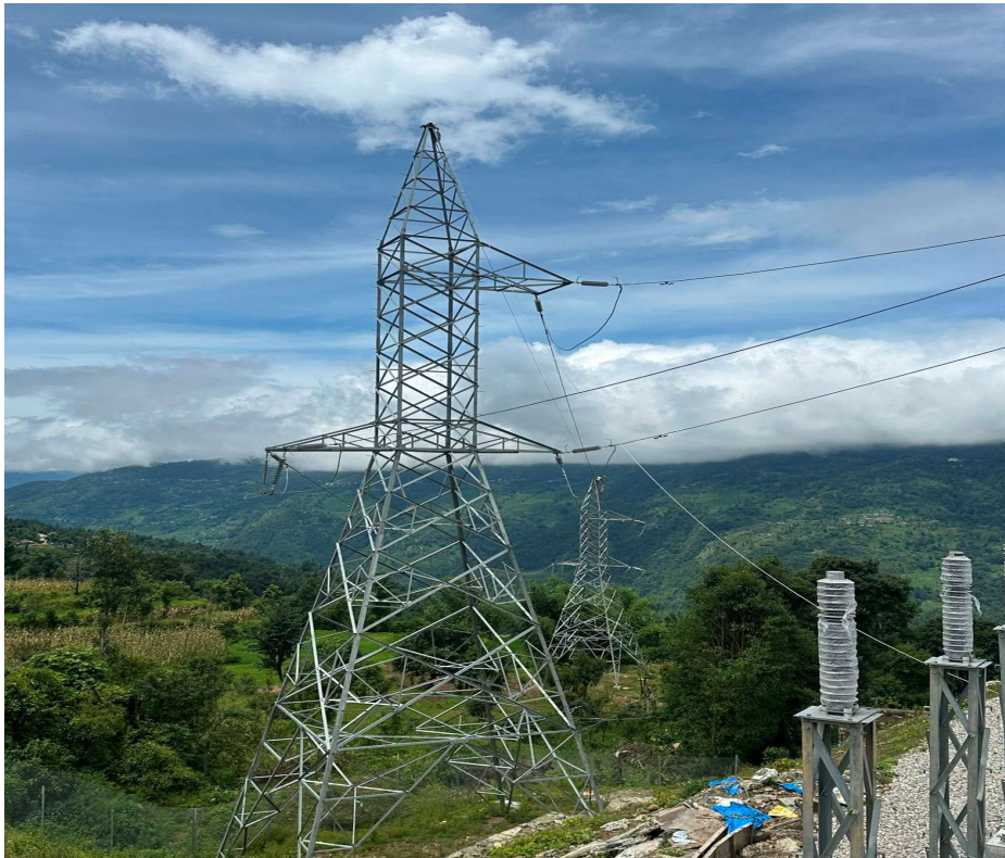
Transmission line conductor stringing
