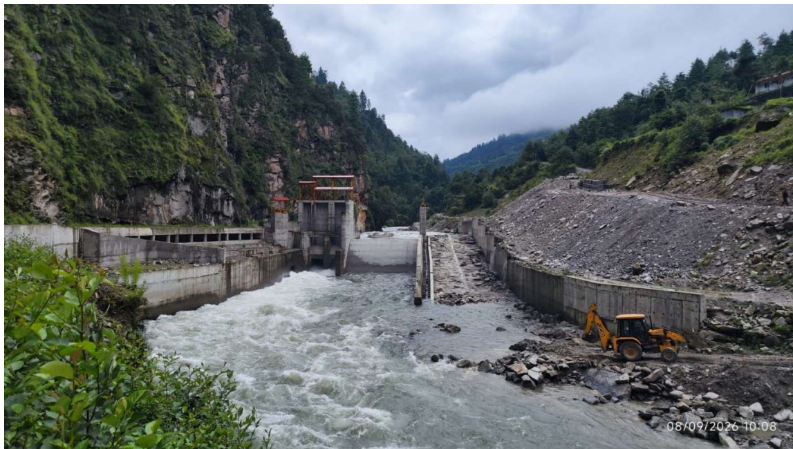
Headworks Structure with Left bank Back fill works continuous
