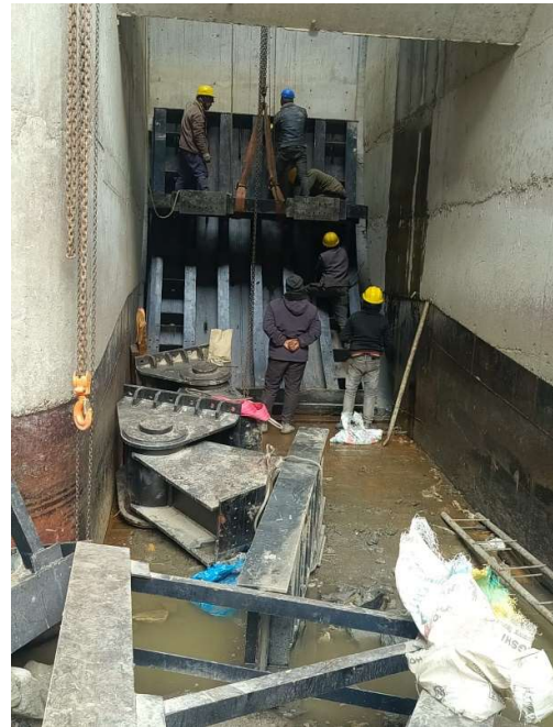
Radial Gate Installation work by HM team
