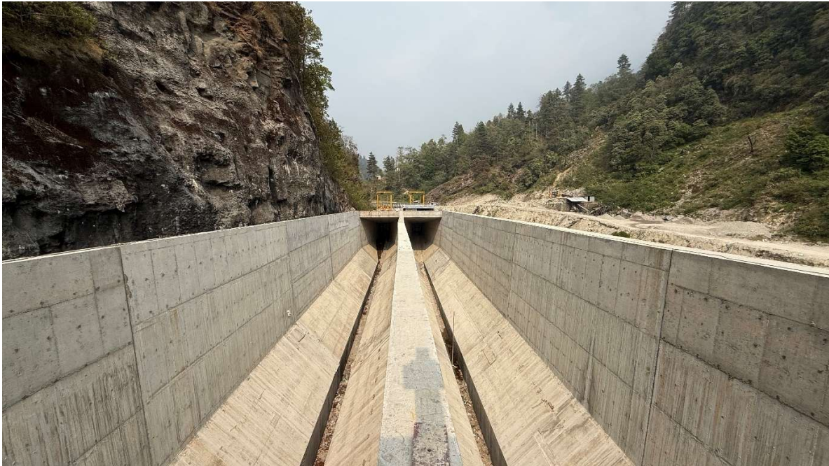
Overall, View of the Settling Basin
