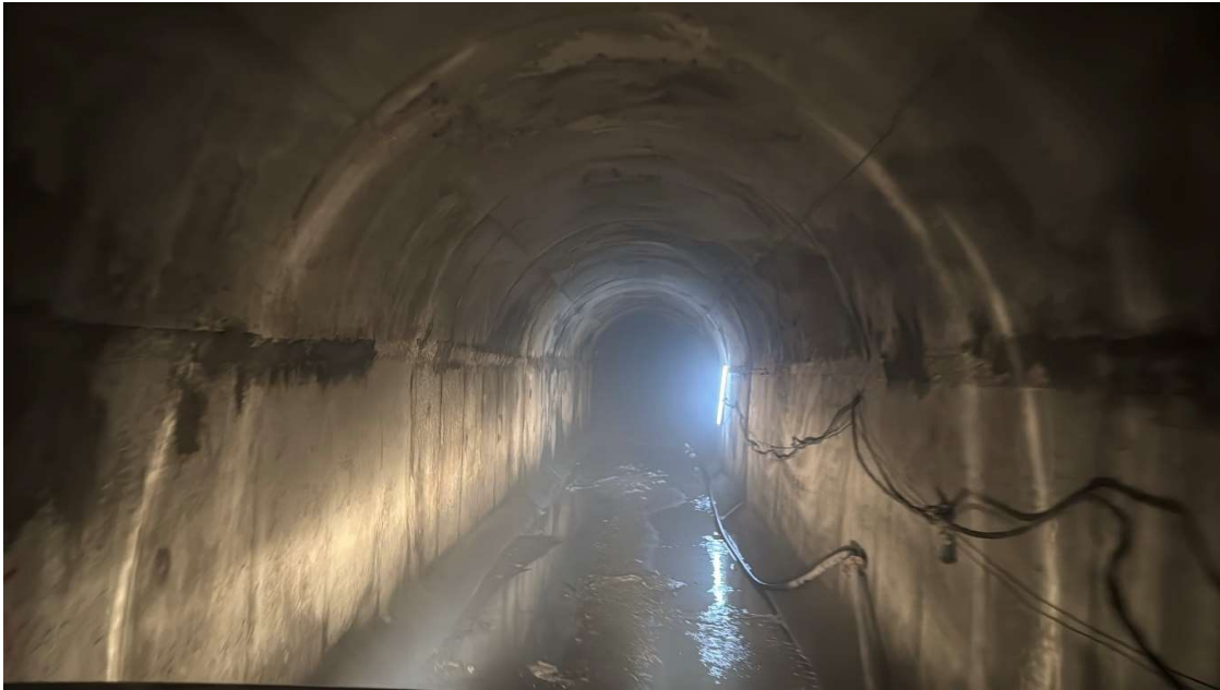
Face 1 Concrete lining work.
