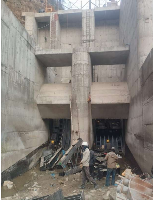
Radial Gate Installation work by HM team
