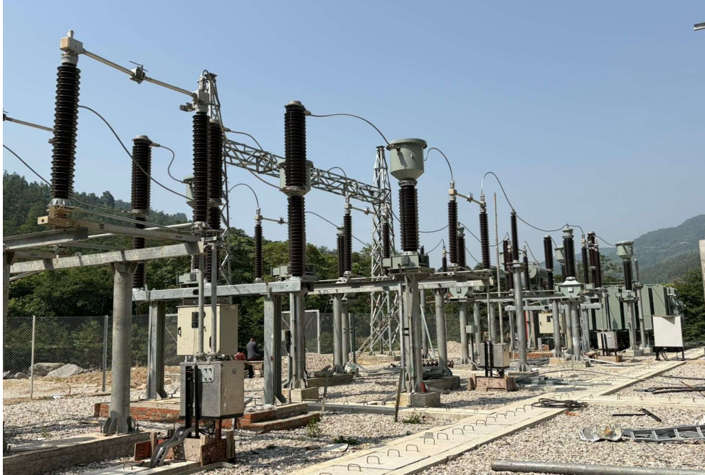
Outdoor 132Kv equipment connection works
