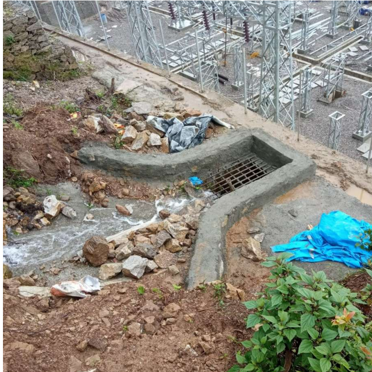
Drainage work at LILO
