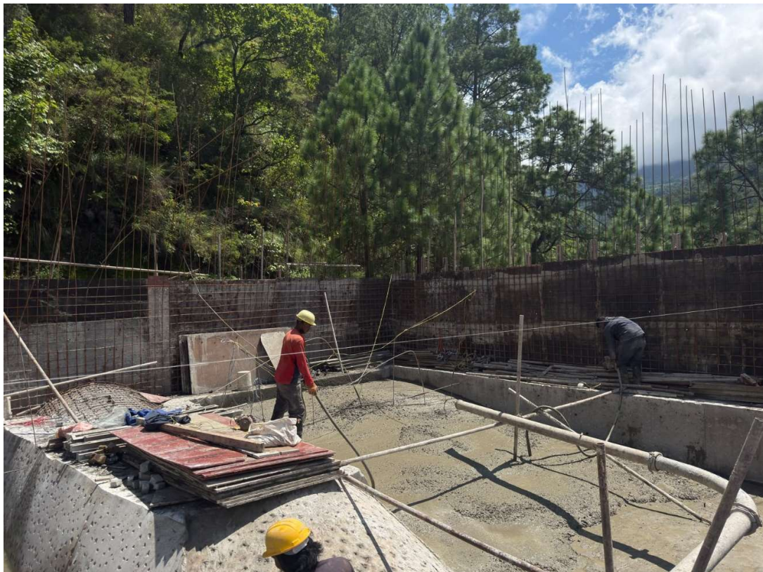
Anchor Block (AB06) Outside of the UPT
