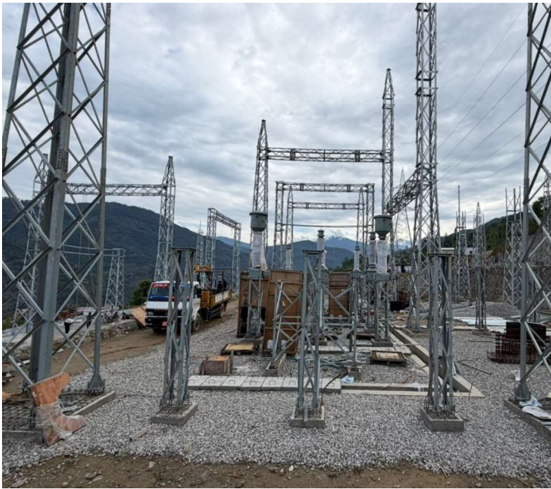
Installation of the Substation EM equipment at LILO by EM team
