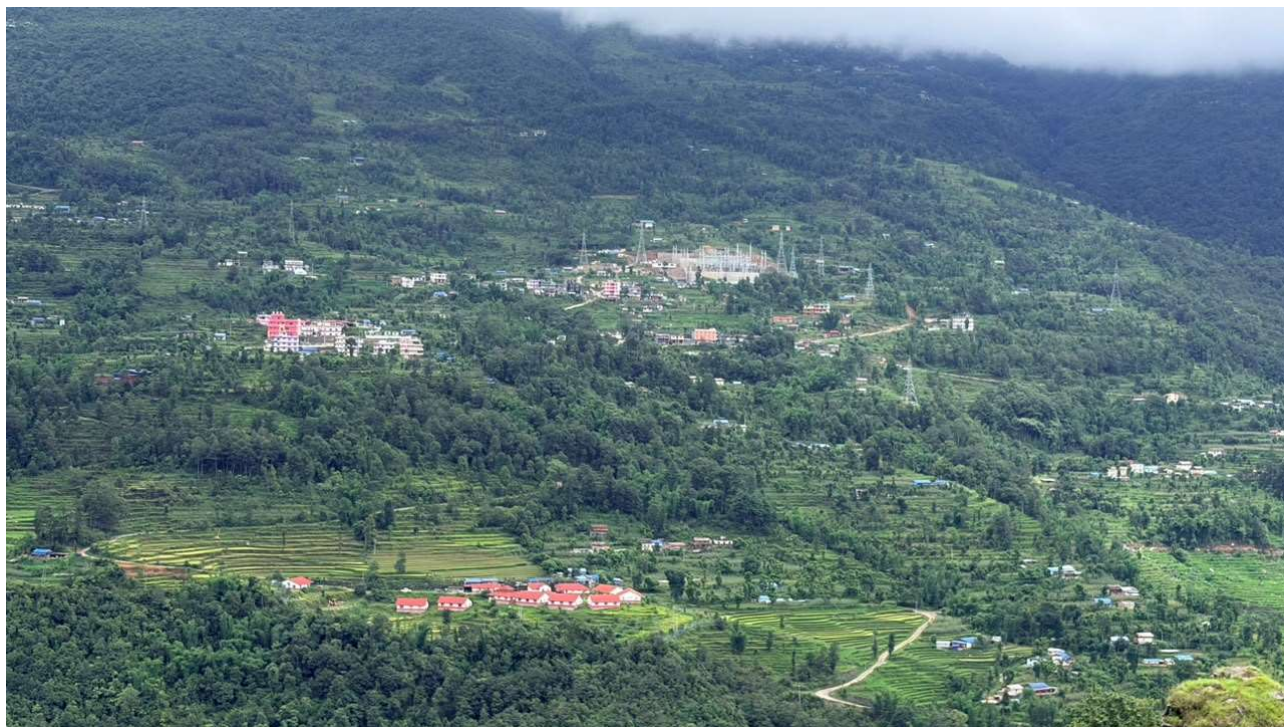
Overall View of LILO
